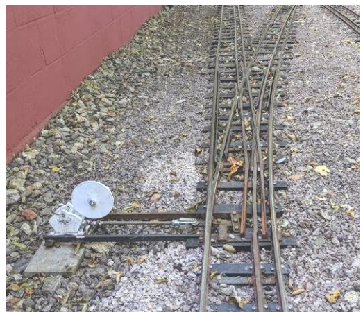
An example of a manual point lever indicating the route set on a facing point.
