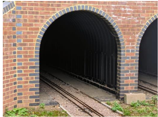
An example of a tunnel portal on a 7¼" gauge railway. Note the headroom and clearances.
